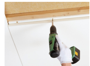
Master F is installed by screw fixing
